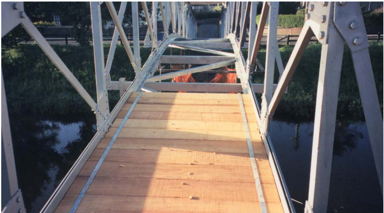
'Near Threatened' 1 African iroko used in the refurbishment of the footbridge over the Grand Canal, Tullamore, Ireland.
